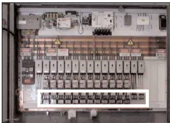
PDB in UL508A, 480V Branch Circuit must have spacing of  $\frac{3}{8}$ " through air and  $\frac{1}{2}$ " over surface. PDBs listed to UL 1953 meet these spacing as well as most terminal blocks recognized to UL 1059.
