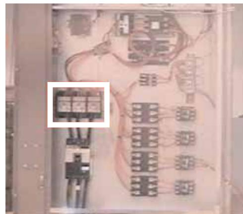
PDB in 480V UL 1995 HVAC Equipment must have spacing of  $\frac{3}{8}$ " through air and  $\frac{1}{2}$ " over surface. PDBs listed to UL 1953 meet this spacing as well as most terminal blocks recognized to UL 1059.
